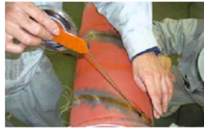
Fig. 3: Fiber installation for long-time monitoring [11]
